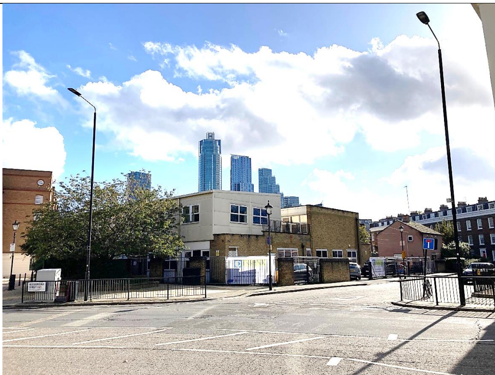
View from Bessborough Street
